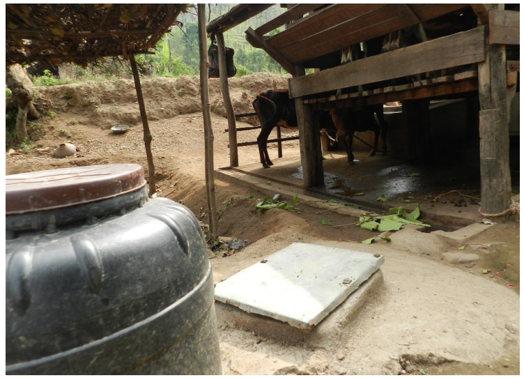
SIFS farm with biogas, cowshed linked with composting unit
