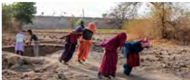
MDG 1: Nimpith: Well construction with the state employment program
