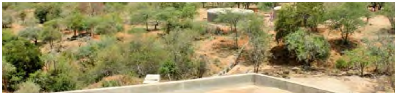
MDG 7: Rain water rock catchment for improved drinking water
